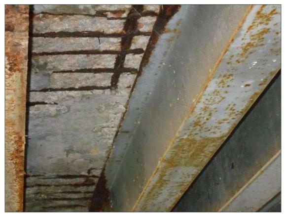
DECK SPALLING UP TO 3/4" DEEP WITH REBAR EXPOSED MIDSPAN BAY 1. SIMILAR NEAR ABUTMENT 1 END BAY1 AND AT BAY 10.
