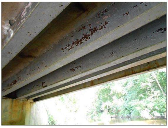
PAINT SCALING AT BEAMS 2 AND 3. SIMILAR AT EACH BEAM.
