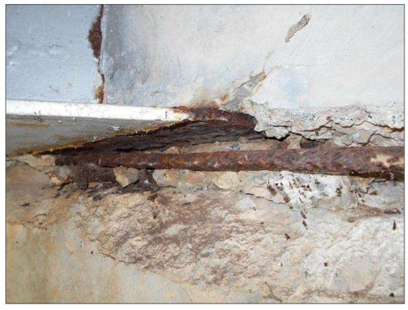
BEAM 10 ABUTMENT 2 END HAS LOSS OF SECTION 3/8" WITH 3/8" SECTION REMAINING IN BOTTOM FLANGE, FULL WIDTH ALONG CAP ENTRY AREA
