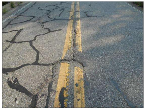
CRACKING IN ASPHALT WEARING SURFACE ALONG CENTERLINE.
