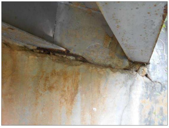
ABUTMENT 2 CAP SPALLING 6' WIDE X 5" HIGH X 2" DEEP WITH REBAR EXPOSED UNDER BEAMS 10 AND 11.
