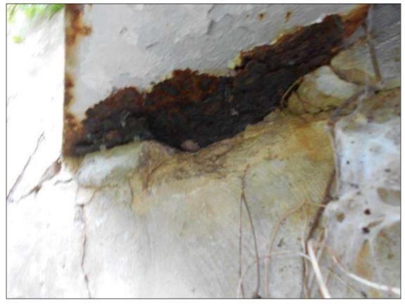
BEAM 11 ABUTMENT 1 END HAS LOSS OF SECTION 1/8" WITH 1/4" REMAINING FULL WIDTH OF BOTTOM FLANGE ALONG BEAM / CAP ENTRY AREA.
