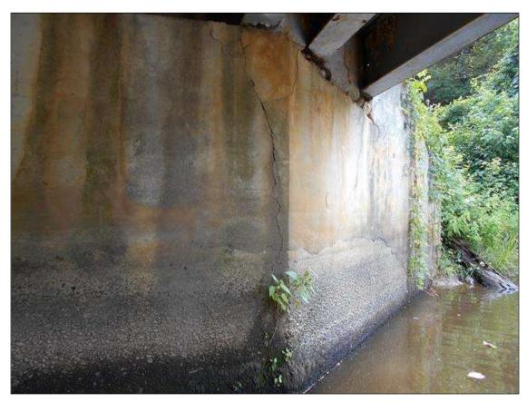
ABUTMENT 2 BREASTWALL HAS VERTICAL CRACKING HAIRLINE TO 1/16" OPEN UNDER BEAM 9.
