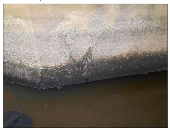
ABUTMENT 2 BREASTWALL VERTICAL CRACKING UP TO 1/8" OPEN UNDER BEAM 3.
