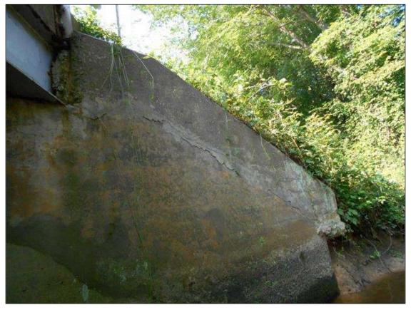
CRACKING ALONG PATCH AT SOUTHWEST WINGWALL
