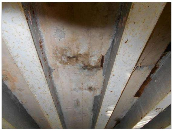
DECK BAY 4 MAP CRACKING WITH DISCOLORATION AT MIDSPAN. SIMILAR AT BAYS 6, 7 AND 8.
