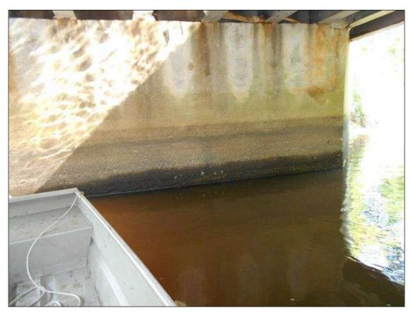
ABUTMENT 1 BREASTWALL HAS COARSE AGGREGATE EXPOSED ALONG BOTTOM 3' TO WATERLINE. SIMILAR AT ABUTMENT 2 BREASTWALL.
