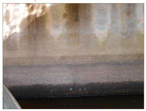
ABUTMENT 1 BREASTWALL HAS VERTICAL HAIRLINE CRACKING UNDER BEAM 5.
