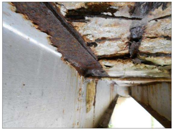
BEAM 10 TOP RIGHT FLANGE HAS LOSS OF SECTION 1/4" WITH 3/16" SECTION REMAINING 4' LONG AT MIDSPAN.
