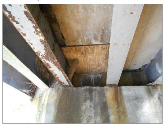
REPAIR FORM IN PLACE AT BAY 8 ABUTMENT 1 END.
